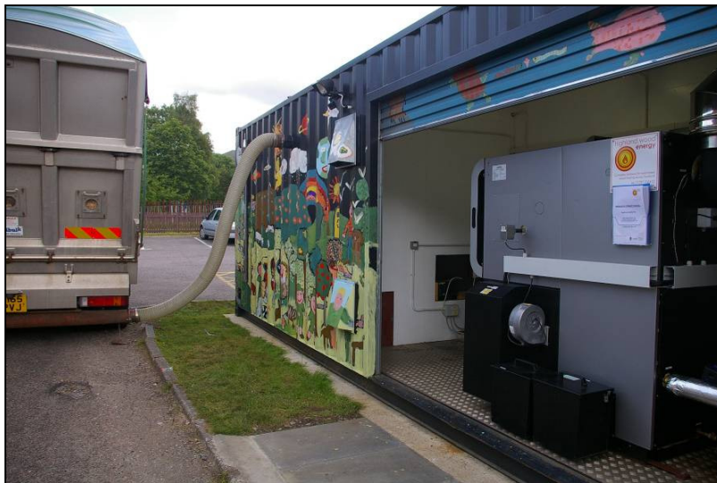
Figure 3.1: Pre plumbed container with wood chip boiler and integral hopper.
