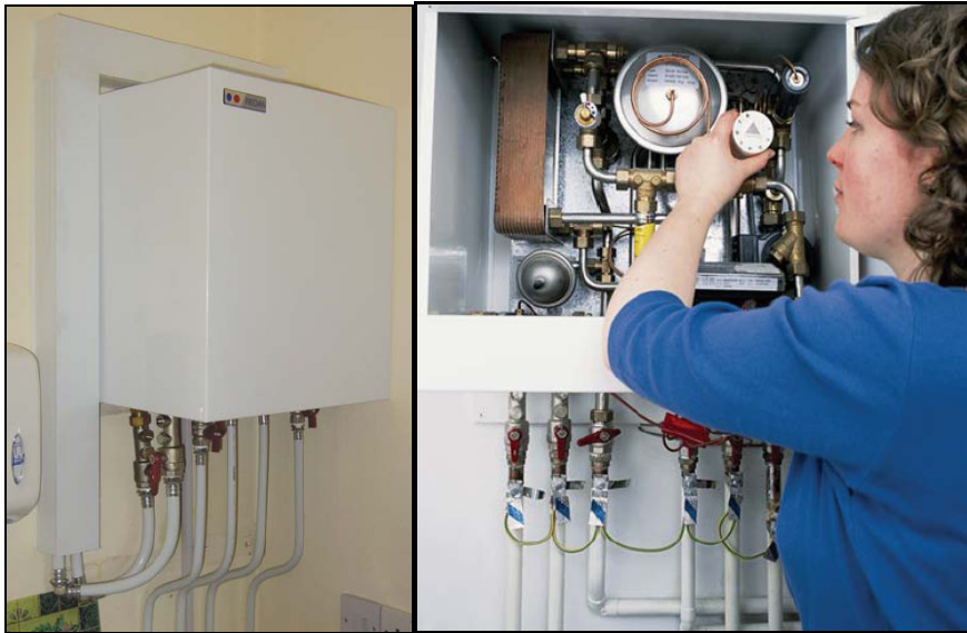
Figure 3.5: Typical Interface Unit (Source: Community Heating – a guide 5 )
