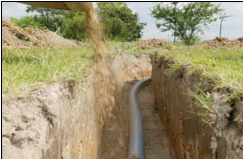
Figure 3.4: Trench for DH pipe
