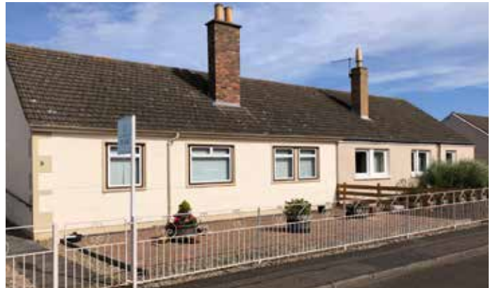
Kirk Brae - home to the right has external wall insulation up to party wall
